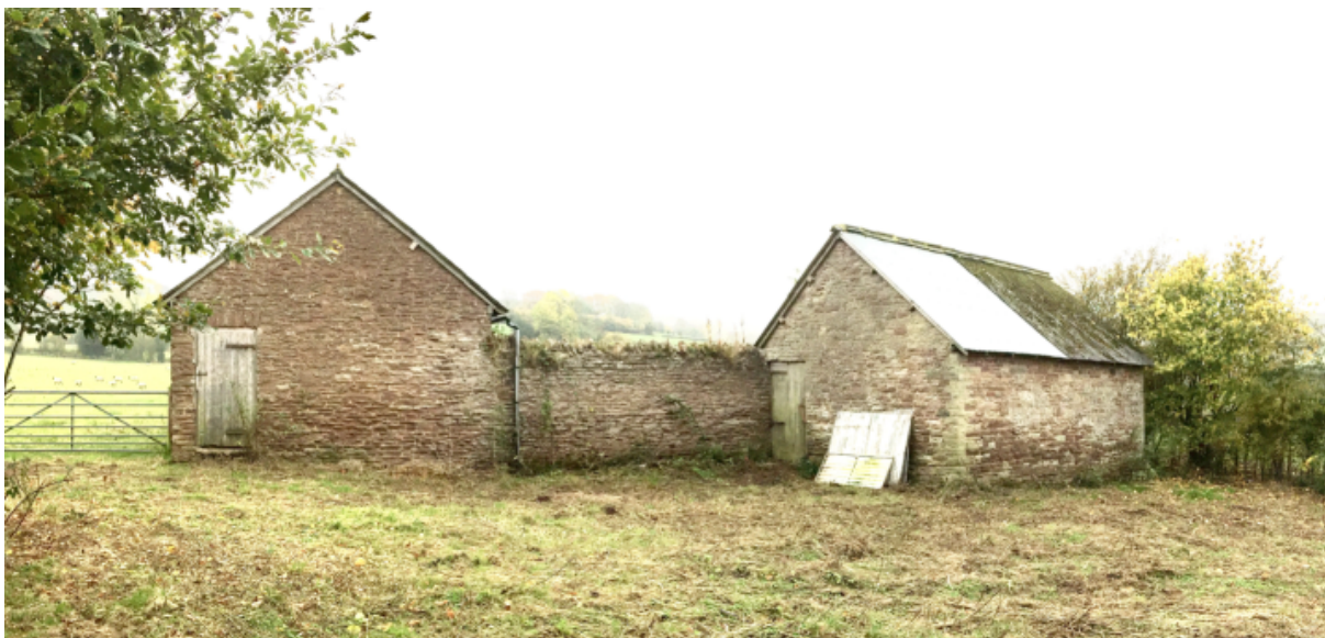
Figs 1 and 2. Main building and outbuilding showing vernacular construction.
